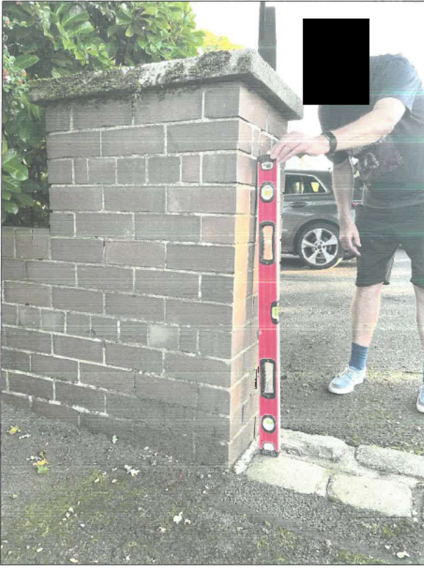
Figure 5. Spirit level showing the lean to the gate pillar.
